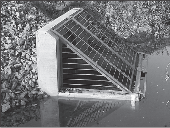
Above: The weir installed at the outlet to Rithet's Bog maintains water levels during dry summer months. Right: Tree Swallows at a nest box installed near the outlet weir. Photo: Bruce Stewart.
